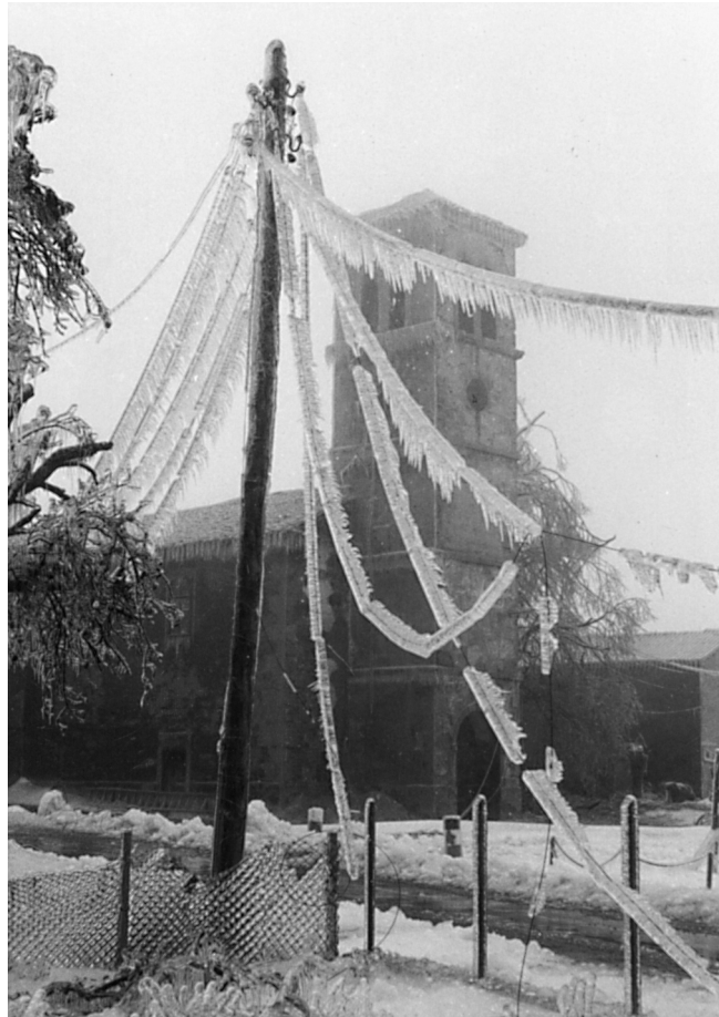
Figure 2. Ice on aerial cables after a freezing-rain event in Slovenia (photograph from IBE, Ljubljana).
